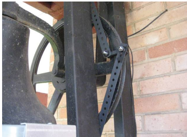
Connect the rope wheel clamp to the perforated steel straps to anchor the bell position to the frame Use Loctite or Gorilla glue on the clamp's threads.
