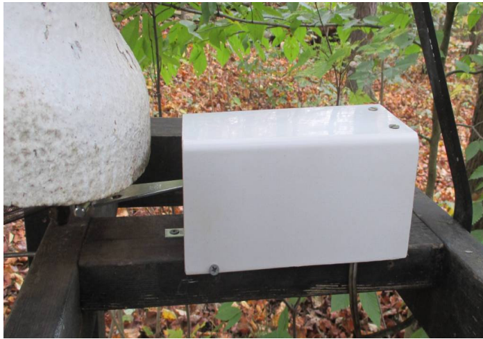
A PVC Solenoid Cover is used for outdoor installations.
